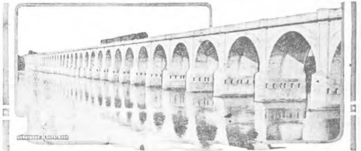
One of the most picturesque concrete arch-type bridges of the country has just been completed across the Susquehanna river at Harrisburg, Pa., by the Reading railroad. It is a double track structure a mile in length and replaces an obsolete bridge of steel.
