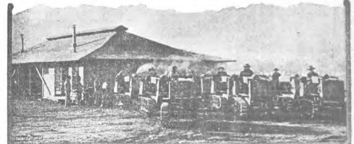
Tanks hauling one of the buildings of the base hospital at Fort Bliss. The base, which was moved to a location some distance away, is one of the most complete in the United States.
