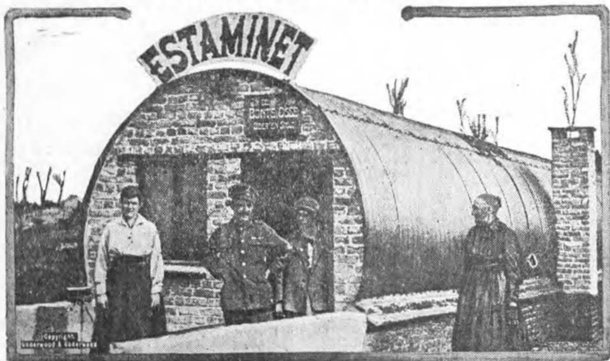
This "estaminet" or cafe at Ypres was built by the Belgian at left of picture. It is constructed of circular strips of corrugated iron salvaged from war dugouts. The proprietor and his wife live in the rear part of the structure.
