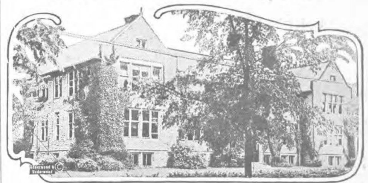
One of the buildings (horticulture) of the college of agriculture, University of Missouri, Columbia, Mo., where the federal board for vocational education has placed disabled world war veterans who desire training in agriculture.
