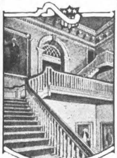
Grand Stairway From the Lobby of the Hall to the Second Floor; the Grand Stair at the Right Above Leads to the Balcony, and into the Belfry; Where the Liberty Bell Originally Hung.
